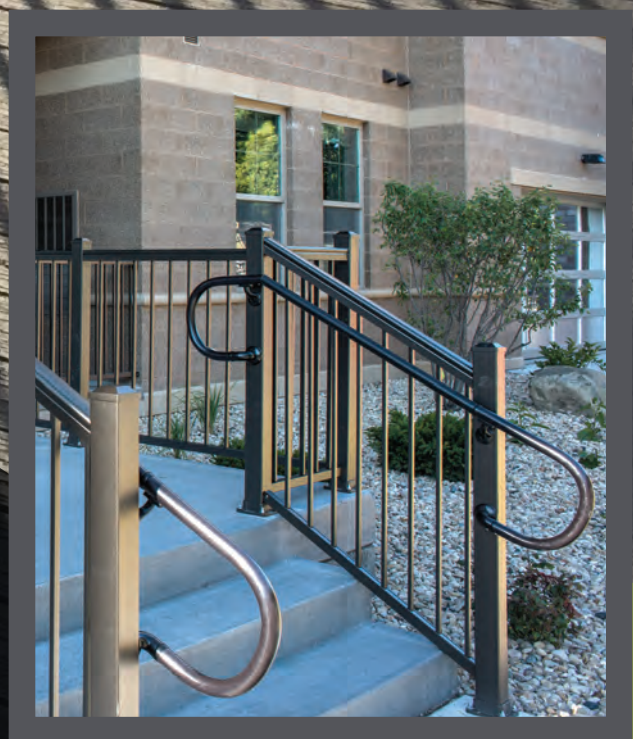
Public Use Ramps & Handrails
